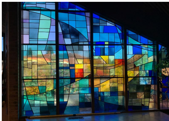
Repaired and cleaned stain glass
